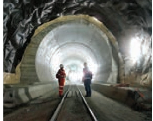
^ The Gotthard Base Tunnel while under construction
